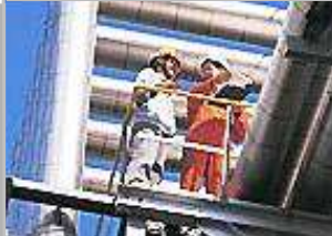
Industrial Process Control
